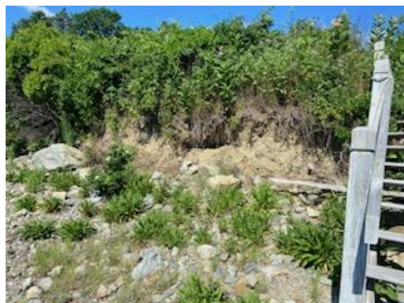
Photo 1 & 2 – Images depicting how the toe of slow has been undercut and compromised.
