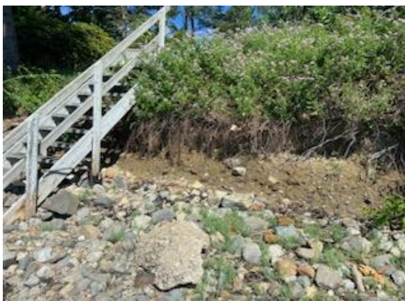
Photo 1 & 2 – Images depicting how the toe of slow has been undercut and compromised.
